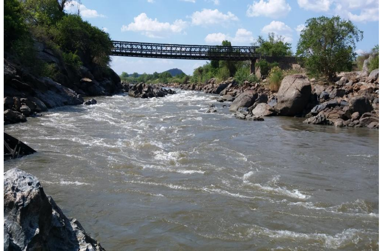
Mpatamanga Hydro Power Project Site
