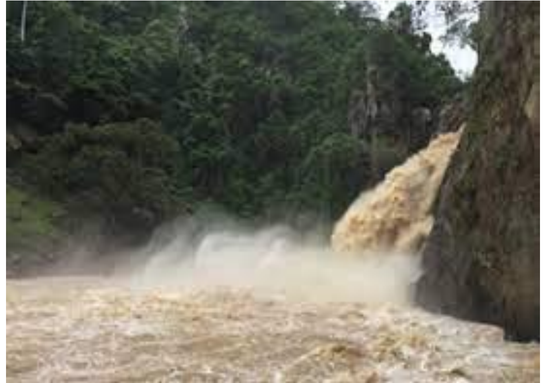
FUFU Hydro Project Site
